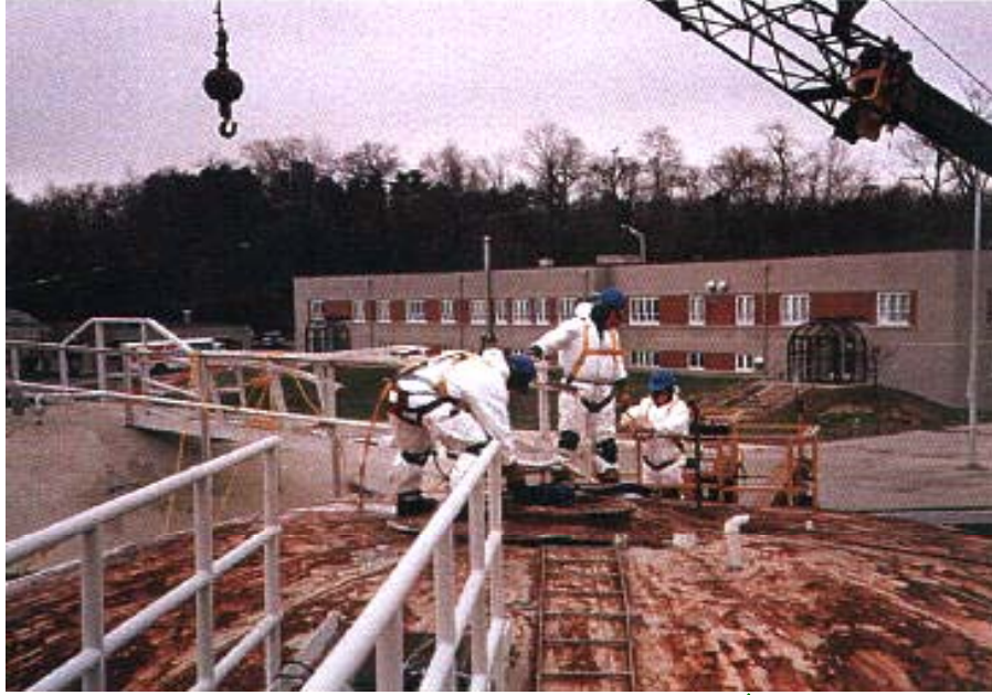
Plant Dismantling and Recycling at Manufacturing Plant ↑
