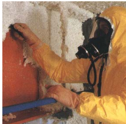
↑Technician Removes Asbestos Fireproofing Material.
