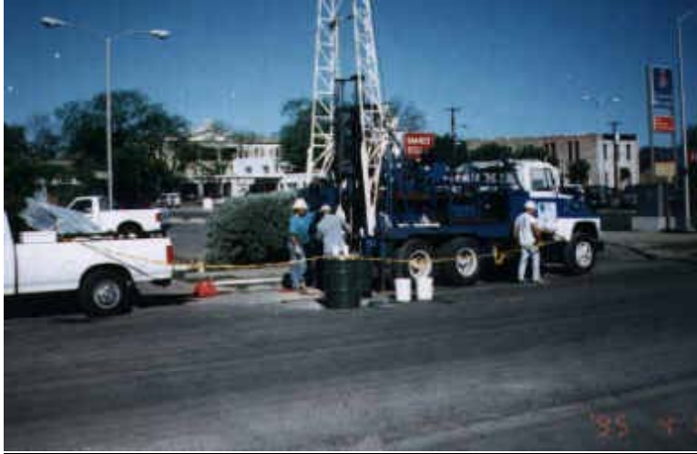
↑ Monitor Well Installation at Chevron Station in Uvalde, TX.
