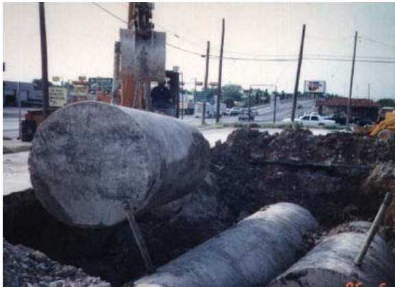
↑UST Removal at H-E-B Grocery Store Site in Del Rio, TX
