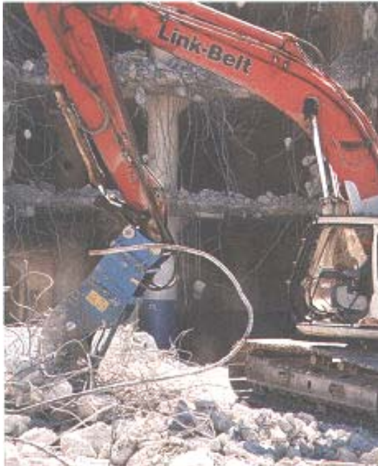
↑Conventional and implosion demolition
